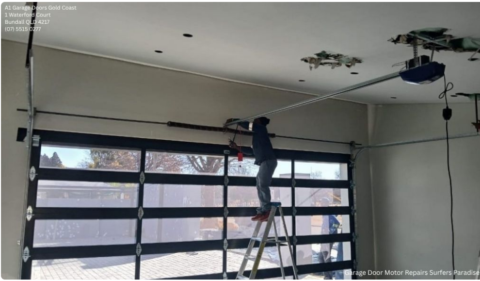
Garage Door Motor Repairs Surfers Paradise
